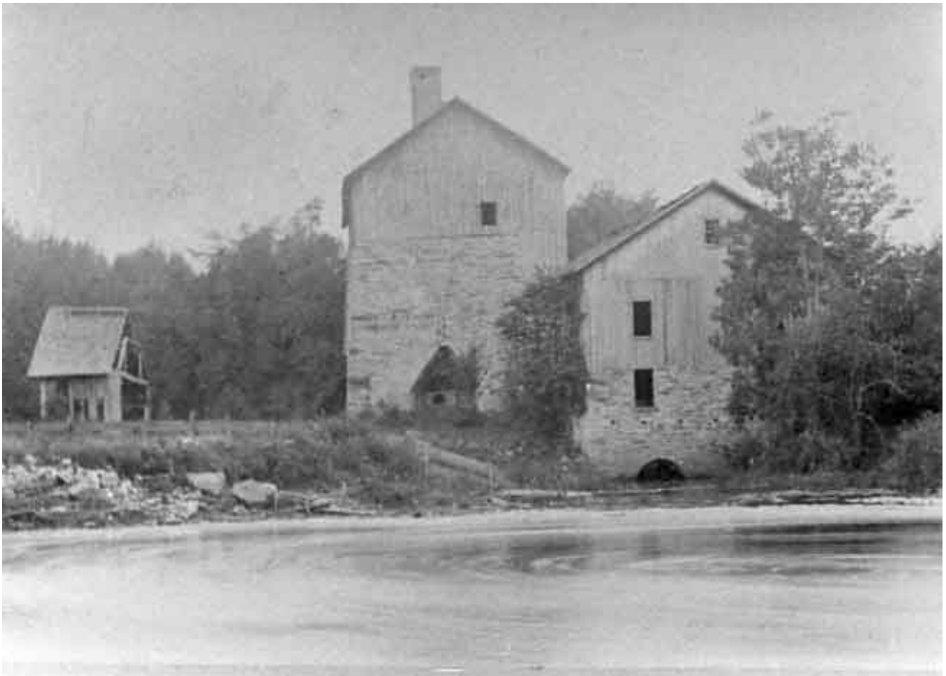
The Grist Mill and Blast Furnace circa 1880
